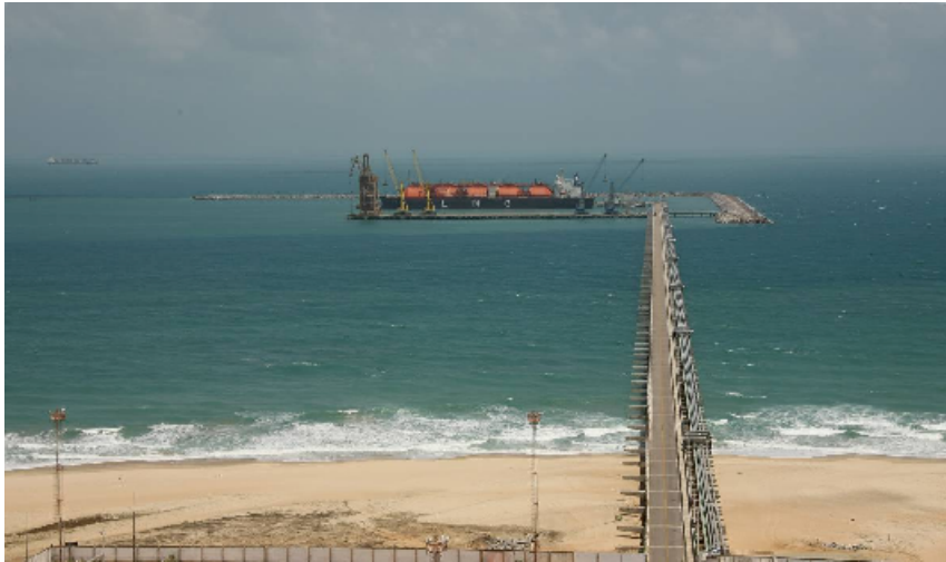
Golar Spirit- Onshore Pipeline View
